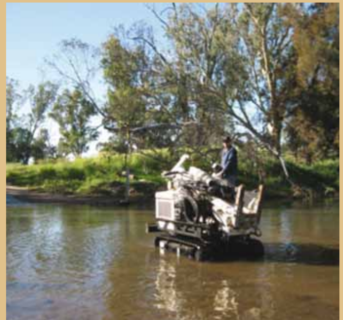
FIGURE 5: Installation of shallow piezometers.
