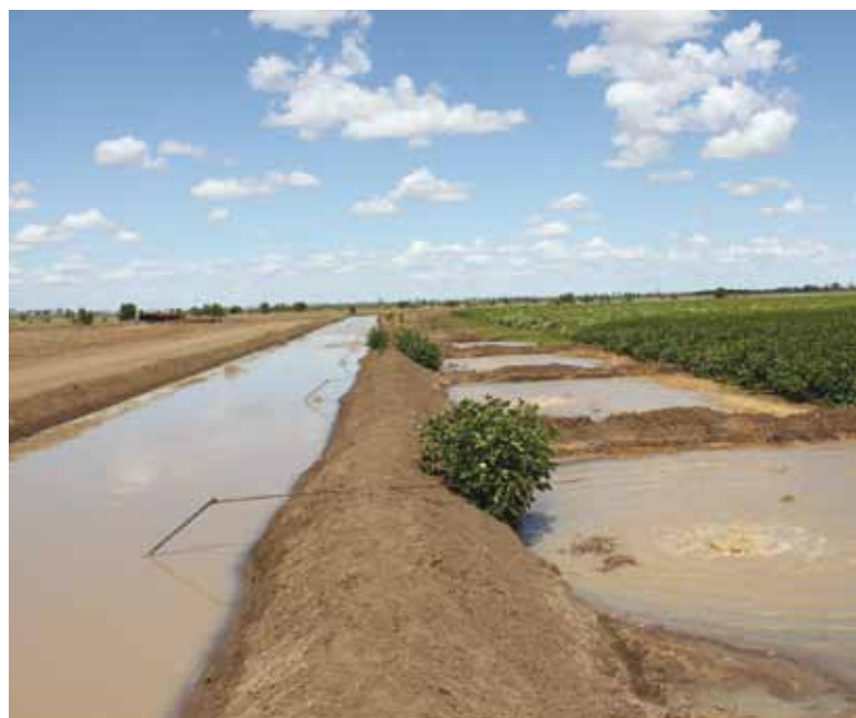
Cotton being irrigated with pipe through the bank system.
