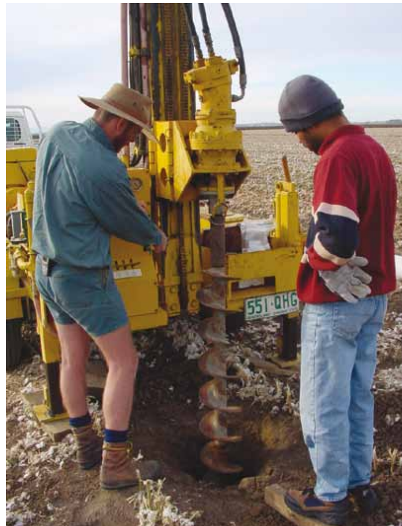
Thusitha Gunawardena (right) installing lysimeters.
